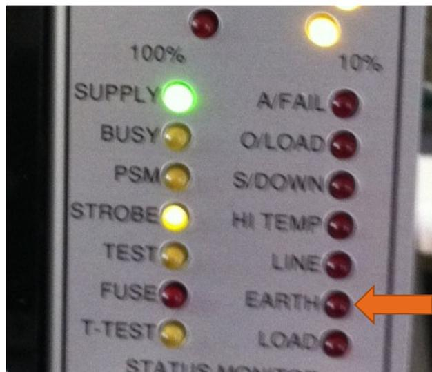
*Earth red LED illuminates whenever earth fault currents are detected from either loudspeaker line conductor and earth.*
