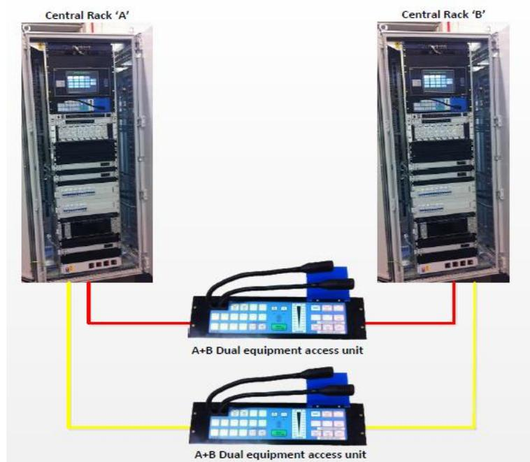
Each A/B system has self-contained resources including independent generation of the site alarm tones. There is no A/B sub system interconnection except for a non-critical optically isolated cable pair (or fibre) between each central rack.
