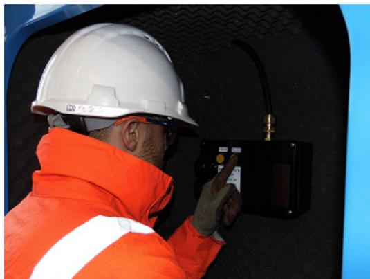
Photo shows ZAP10-02 Ex intercom/PAGA noise cancelling access unit fitted in an AH23-60079 Zitzel acoustic hood, keys are large enough to be operated with gloved hand, duplicated circuits for mission critical application.
