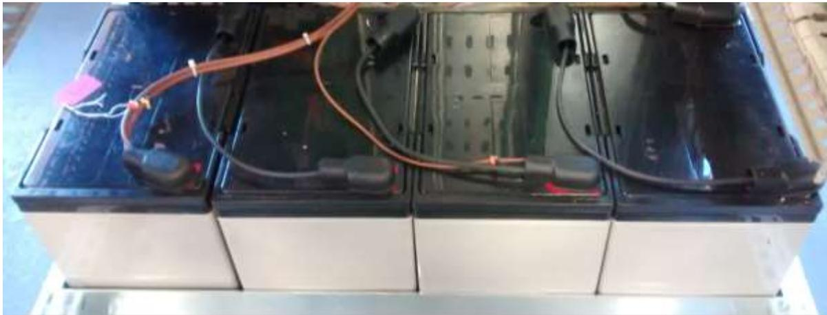
***Target VRLA lead acid battery pile delivers no break 48 VDC secure supply to host equipment rack power consumers.***
