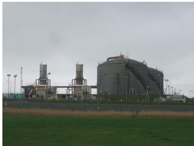
Cruden Bay Terminal Scotland, part of the BP Forties field pipe line installation. This was fitted with one of the first CCE PAGA systems designed by John Blach in the 1970s
